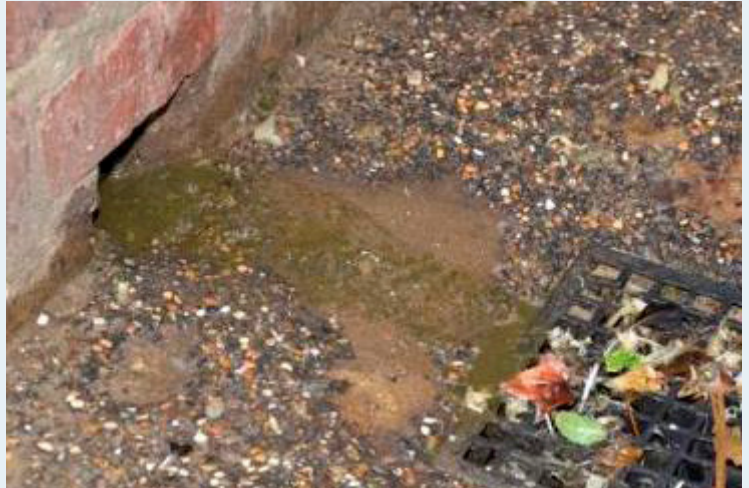
Do not allow run-off to contaminate walkways
